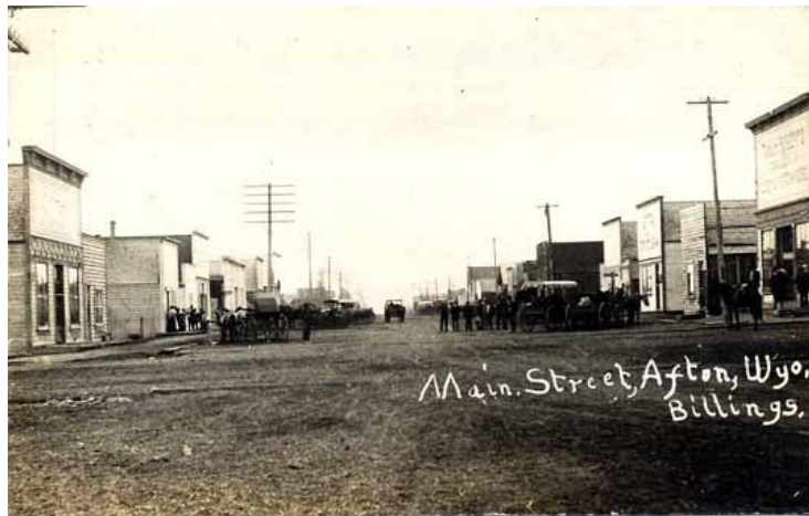
Afton Main Street about 1920 after Telephones came to town (Wyoming Tales and Trails).
