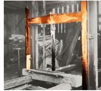
Up-down (or Sash-type) Sawmill.
