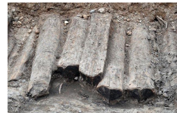
A corduroy road or log road is made by placing logs over a low or swampy area. Impassable mud or dirt roads are improved, but still a hazard (The Record, UofWaterloo).
