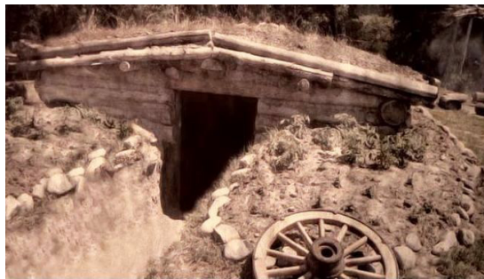
A pioneer dugout with sod roof preserved in Utah, similar to those in Goshen (Utah State Parks, utah.gov).
